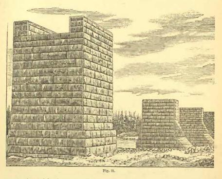
connection with the embankment. It also shows a common form of pier adopted in cases where the structure is opposed to running ice.
